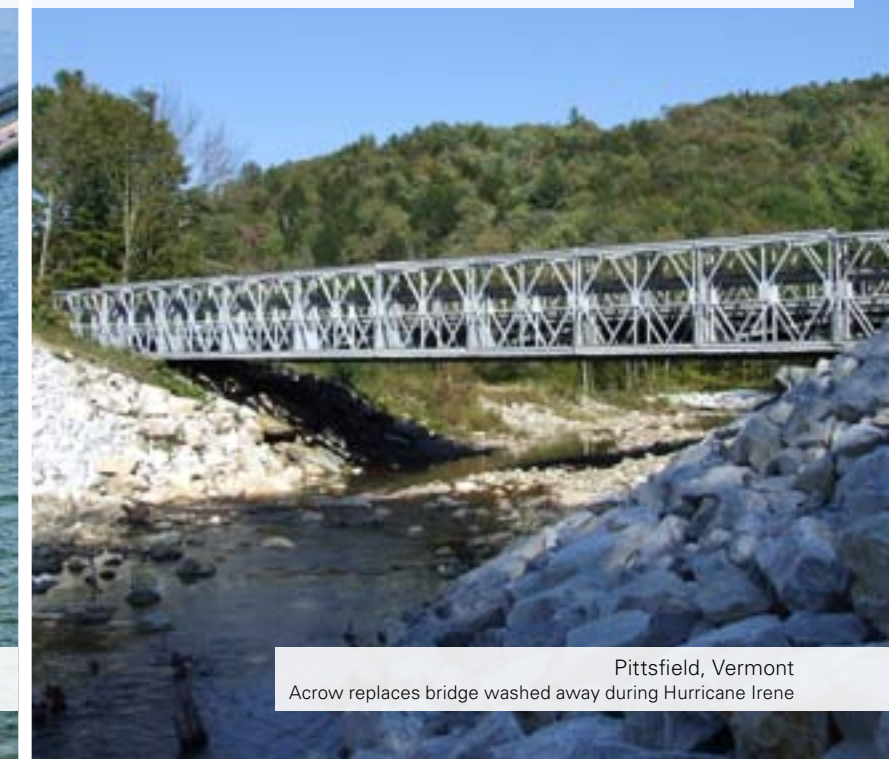
New Orleans, Louisiana Acrow restores major causeway lost to Hurricane Katrina
